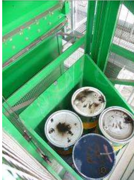
Drums Being Lifted to Shredder
