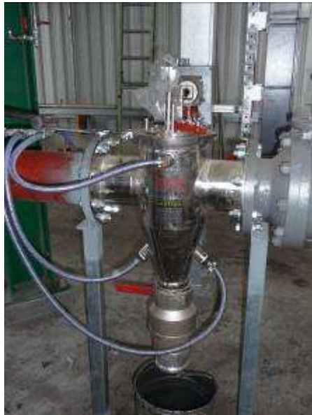
Superblender Fuel Outlet Magnetic Trap
